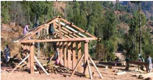
Conventional reconstruction from timber
