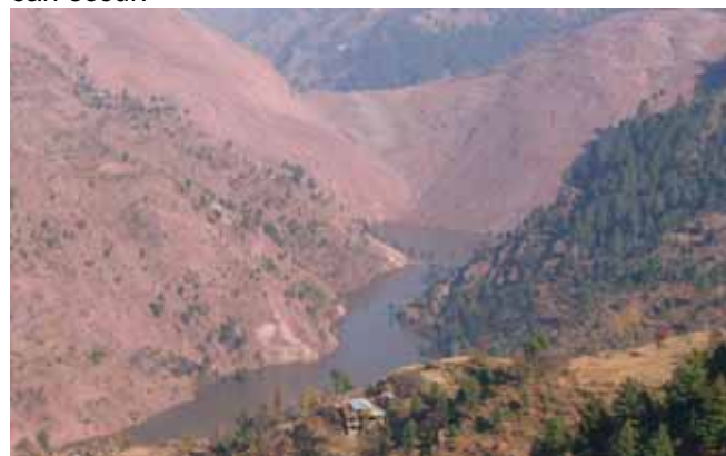
Landslide between Hattian Bala and Chakaar blocking the river
